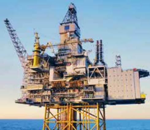
Oil & Gas Pipe Line
